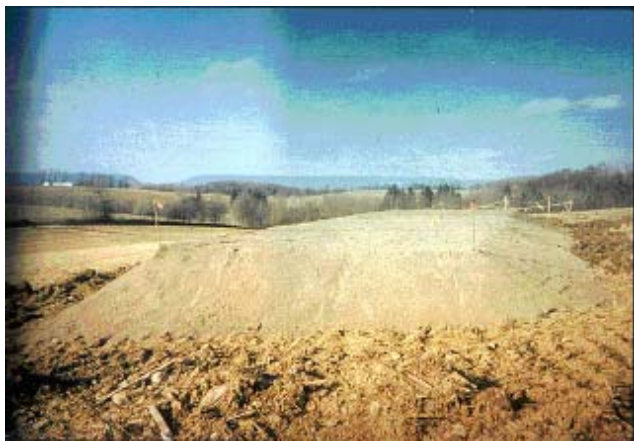
Figure 6. Elevated sand mound under construction.
