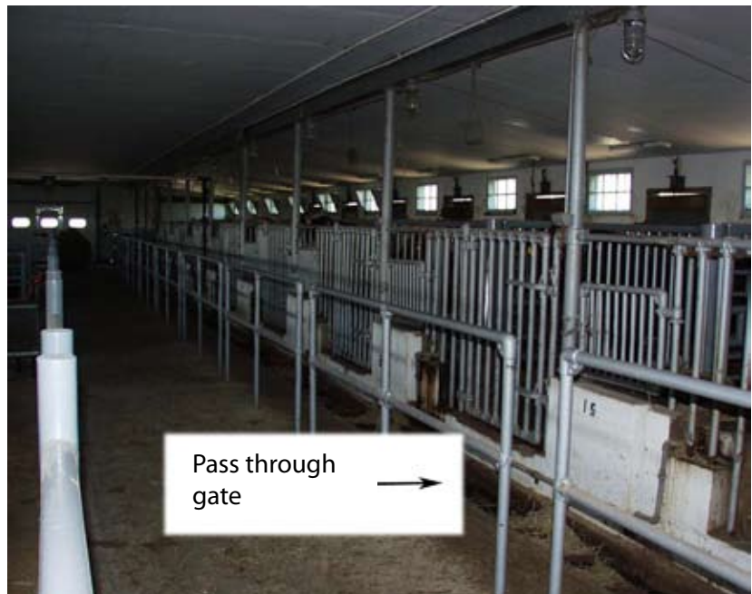
Figure 3. A pass through gate provides an "escape path" to allow a person to move quickly away from an animal.
